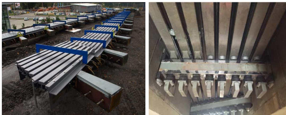
Fig. 2: Examples of expansion joint in bridge along Silesian motorway A1 Gliwice - Ostrava
