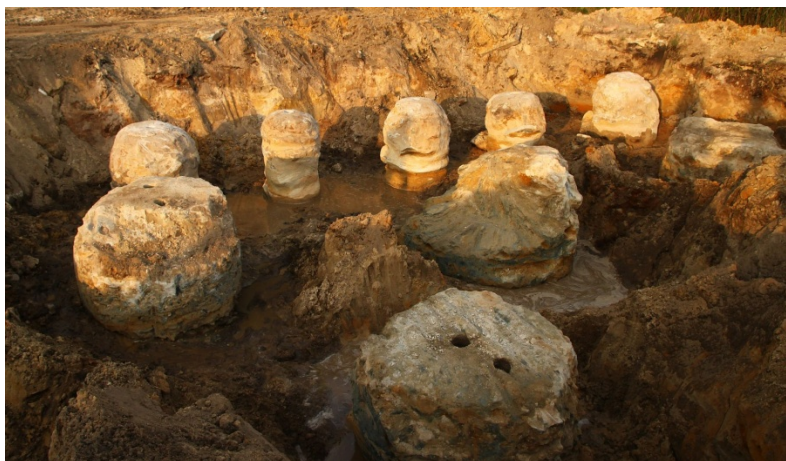
Fig.2: Excavated jet grouting columns (own photos)
