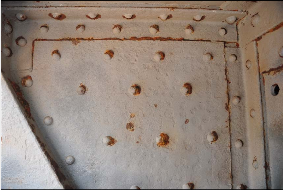
Fig. 5: Pitting corrosion of a steel plate.
