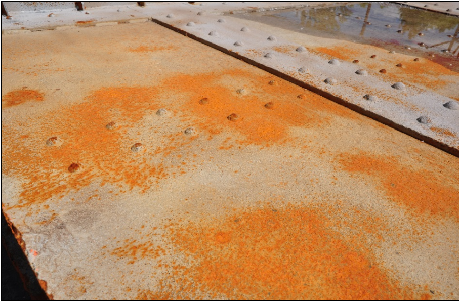
Fig. 4: Deterioration of a steel cover plate.
