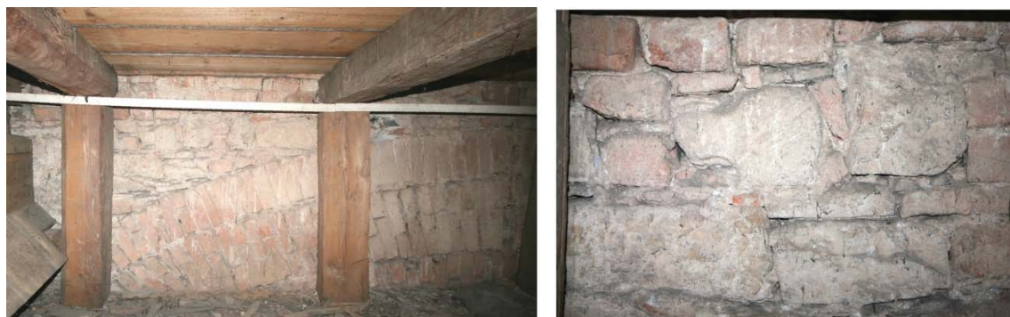
Fig. 27, 28: Southwest side of the church, brick supporting arch above medieval wall and reused masonry above, visible in the space below the upper floor, photograph, 2016.
