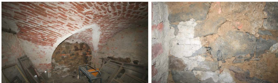
Fig. 35, 36: Partially submerged main floor, Early Modern brick vault and medieval peripheral walls with remains of plaster containing clay and organic material, photograph, 2015.
