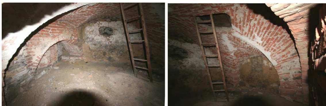
Fig. 37, 38: Partially submerged main floor with medieval peripheral walls and brick vaults, photograph, 2015.
