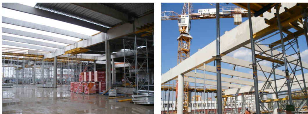
Fig.1: Pre-stressed roof purlin in real structure
