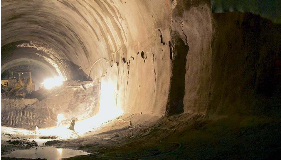
Photo 1: Photo from the point of origin of the collapse - shear failure in the right side of the lining
