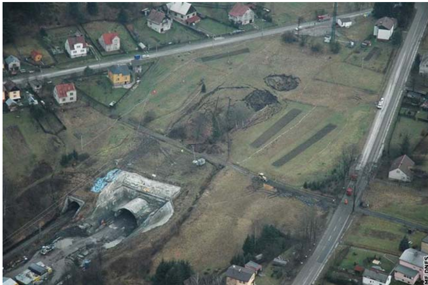
Photo 2: Photo from the point of the origin collapse - formation of the surface crater (author MF Dnes)
