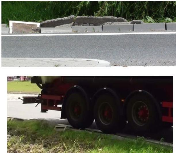
Fig. 4 Details of the damaged kerb at the A exit and a trailer train driving too close to the kerb
