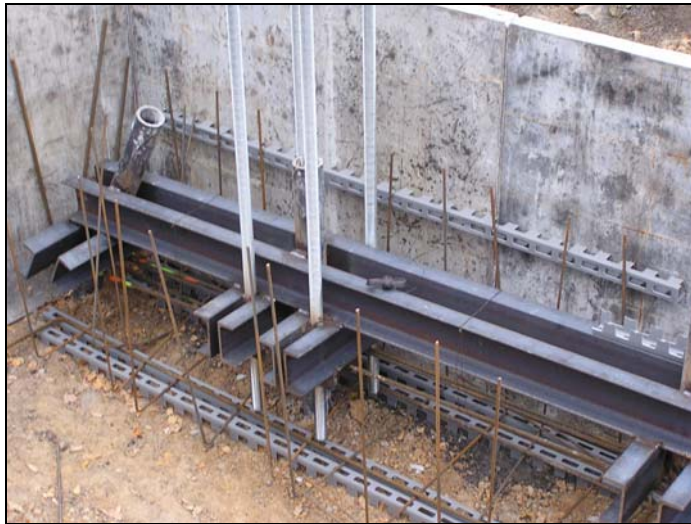
Fig. 4: Detail of the continuous strip footing, anchoring grate and micropiles
