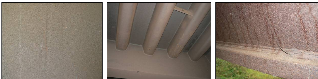
Fig. 2: Appearance of the patina on the indirectly wetted surfaces (left – patina on the web of the main girder in a road bridge in Frýdek-Místek, middle – patina on the orthotropic bridge deck in a road bridge in Ostrava, right – patina on the web and lower flange plate in a highway bridge across the Odra River in Ostrava)
