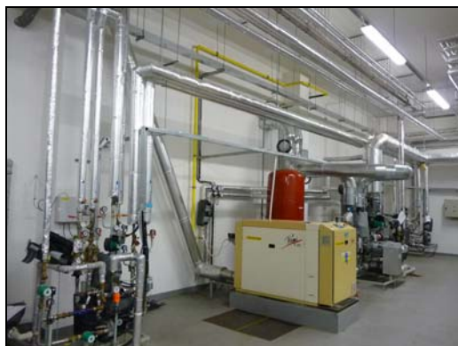
Fig. 6: The cogeneration unit [9]
