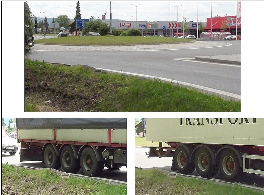
Figure 1: Roundabout Masarykova – parking Tesco in Valašské Meziříčí (up) and detailed views of exit guide strip (down)
