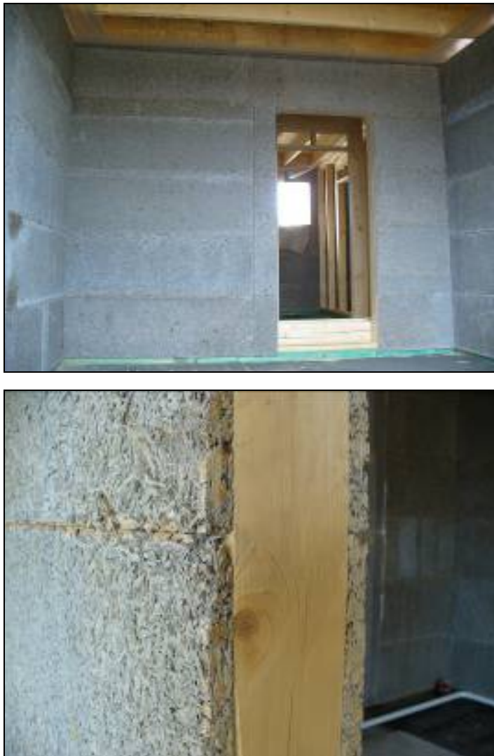
Fig. 1, 2: The usage of VELOX boards as a wall-cladding of wooden structures with the wooden frame
