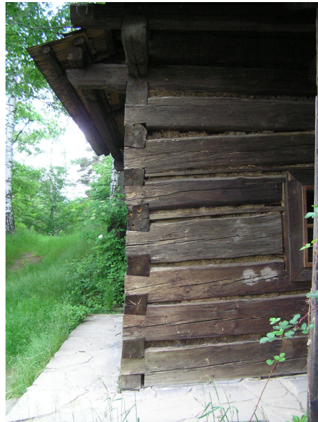
Fig. 6: A vertical corner in external made from timber logs
