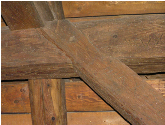
Fig. 5: A complex timber joint
