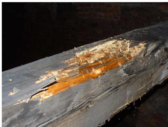
Fig. 1: A wooden component attacked by a house longhorn beetle
