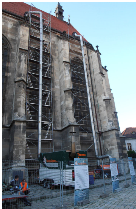
Fig. 2: Hot air heaters and distribution pipes
