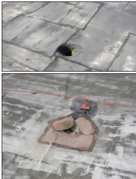
Fig. 1 and 2: Examples of defect implementation of a drain in a roof detail
