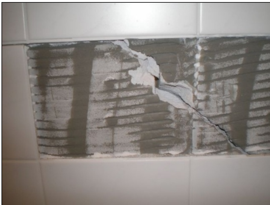
Fig. 3: A common defect – breaches in the partition construction
