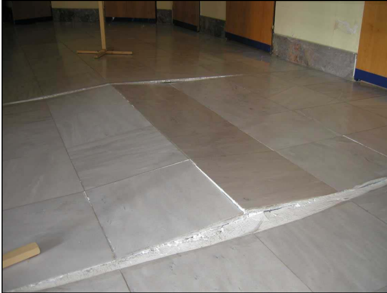
Figure 1: Deformation of the floor and tiles
