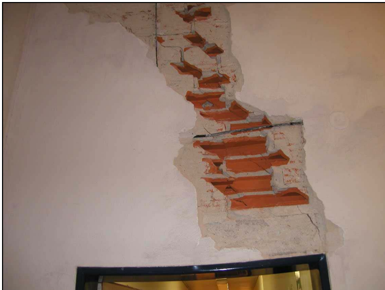
Figure 2: View of damaged brickwork of the non-load bearing wall
