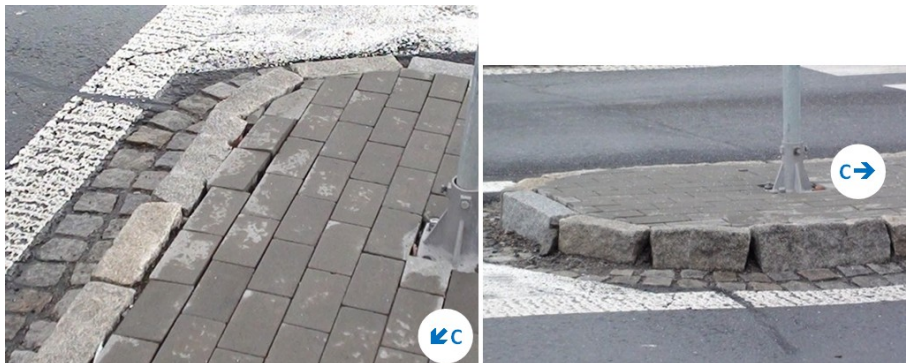
Fig. 11: The damage curb of refuge island on leg C
