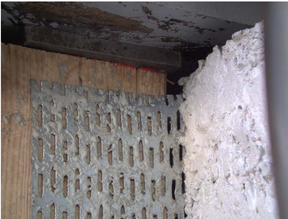
Fig. 4: Slope of gangnail
