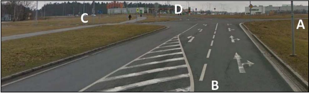
Fig. 3: Sight of intersection from leg B (traffic lane widths 3.00 m, running lane width 3.25 m, guide strips 0.50 m, right corner – compound horizontal curve with radii 30.00 m and 4.00 m)
