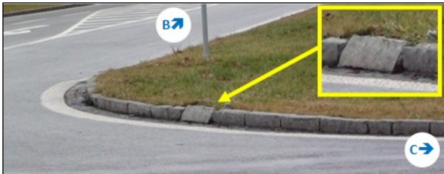
Fig. 9: The damaged curb of corner (from C to B)
