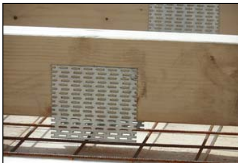
Fig. 1: Detail of coupling of timber and concrete
