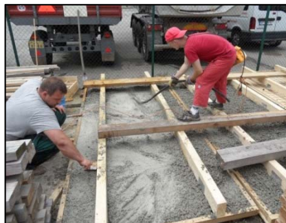
Fig. 2: Concreting of panels
