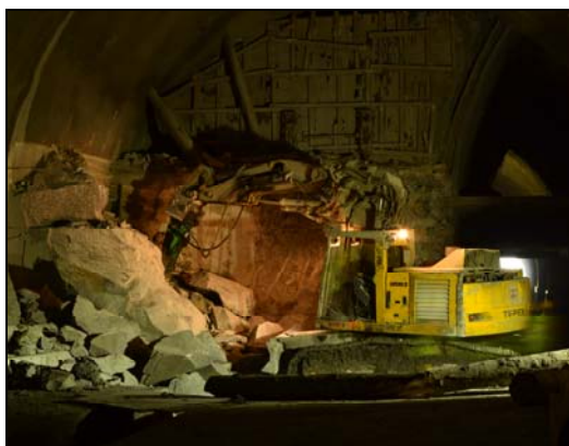
Fig. 1: Heavy crawler excavator TEREX TC 240
