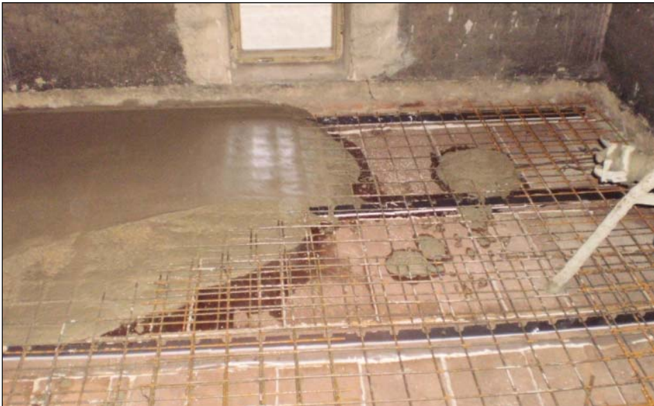
Fig. 8: Concreting of reinforced concrete slab coupled with timber beams
