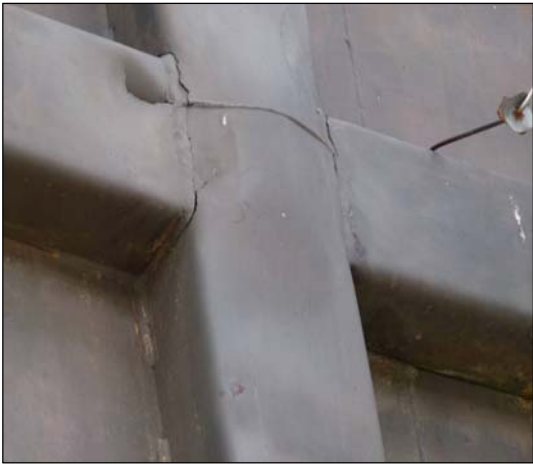
Fig. 4: Cracks at the stiffeners crossing
