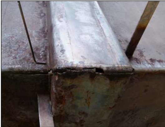
Fig. 3: Cracks in stiffeners at the corner
