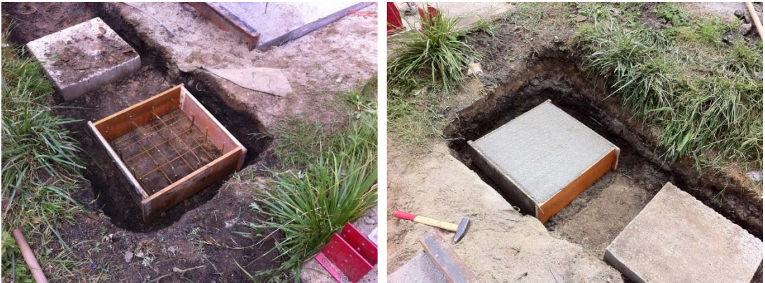
Fig. 3: Realization of base slab
