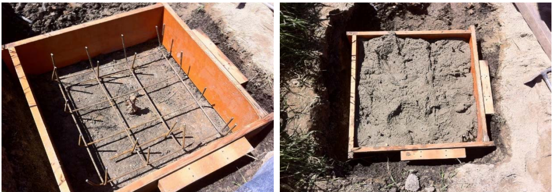
Fig. 2: Realization of the concrete slab above the pile
