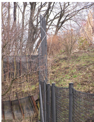
Fig. 9: Bent fence in the top part of the slope deformation (left) Figure 10 Terrain deformation with the manifestation of floor bulging in the workshop up to 15 cm (right)
