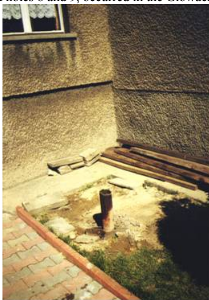
Fig.7 Filling in the underground cavern in the area of sinks 7
